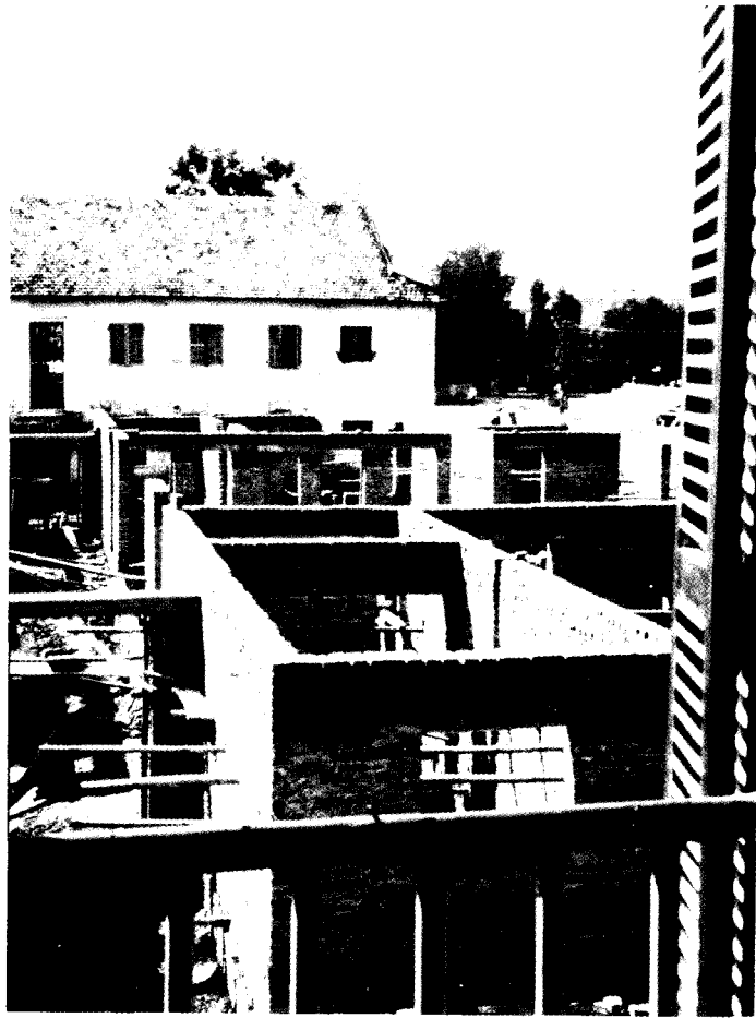
Plate 5. The extension under construction.
