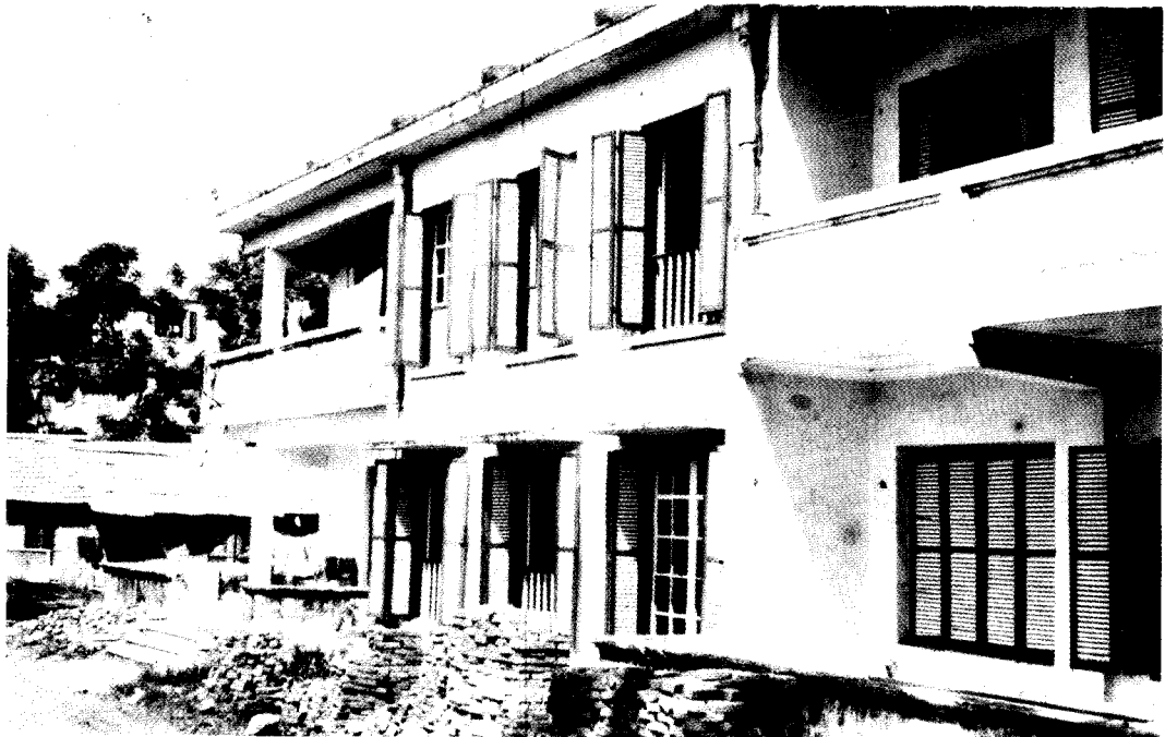
Plate 6. The existing two-storey building.
